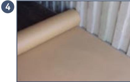
4 Roll out ABSORLINER on one side of container floor and cut to length.
