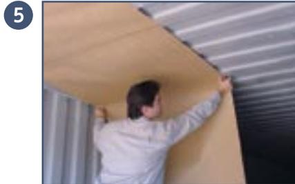
5 Attach ABSORLINER to one side of the ceiling. Start at nose of container and work to doors.
