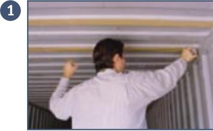
1 Apply adhesive transfer tape on every 4th roof rib across the width of the container. Make sure the area to be taped is free from dust and other contaminants so that adhesive tape will stick.
