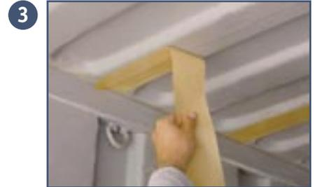
3 Remove tape liner to expose the adhesive film.
